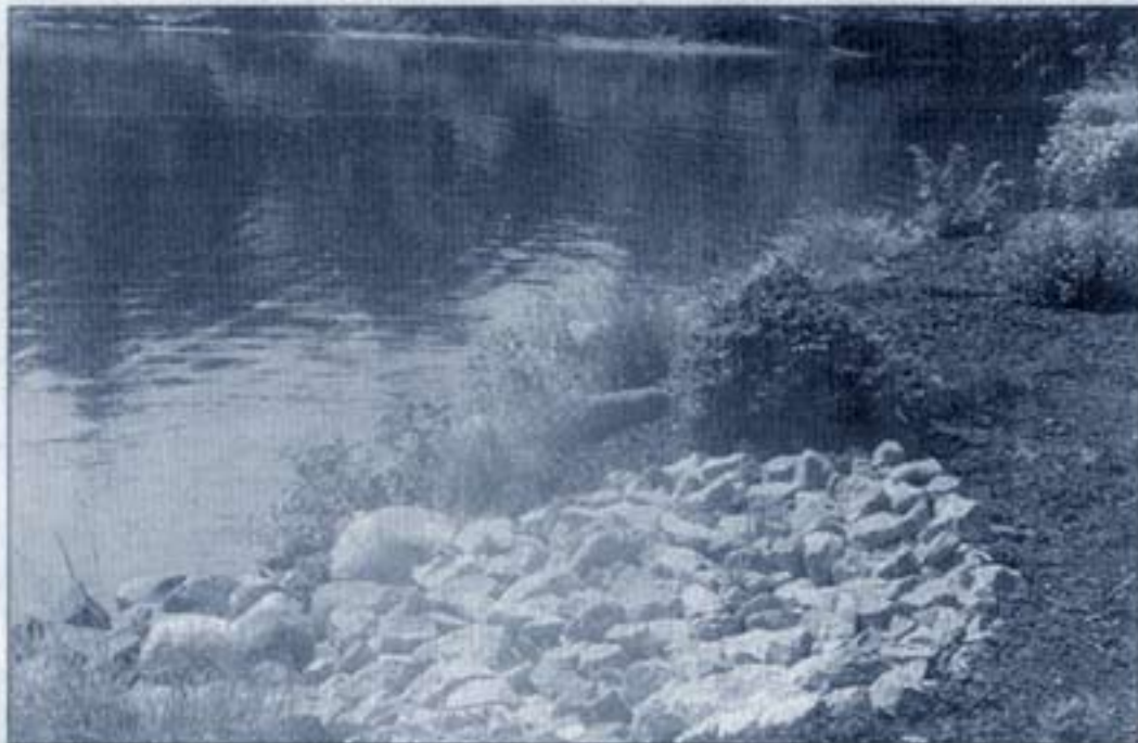
A smaller washed-out area was also filled in with granite stones to prevent further erosion by Lake Maranacook.
