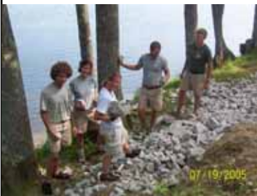
2005 Program Director Crystal Hitchings installing rip-rap with AmeriCorps members.
